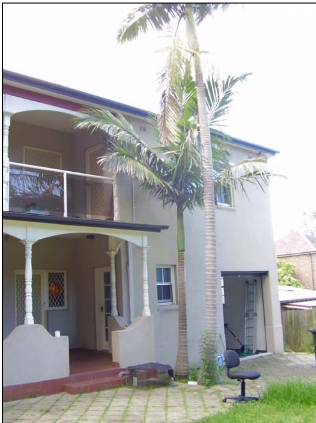
Figure 3.35 The rear of the building. The garage extends through the ground floor of the rear wing. An opening is located at the eastern end.
