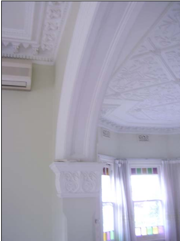
Figure 3.46 The wide arch and details between the two main ground floor rooms.
