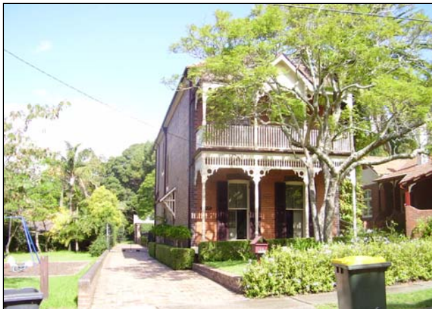
Figure 3.9 No. 14 Wyatt Avenue is a two storey face brick Federation period dwelling with slated roof and prominent front verandah and balcony with timber details. The building is highly intact and is sited relatively close to the street frontage and is enhanced by its front garden setting.
