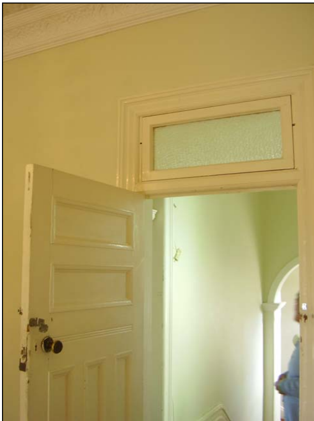
Figure 3.51 The main wing generally retains original timber joinery including timber panelled doors and toplights also architraves and skirtings.
