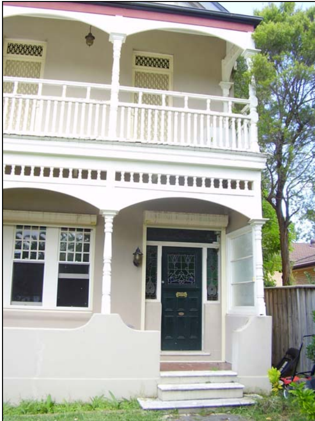
Figure 3.41 The main building entry retains the original timber and leaded glass panelled door, side and toplights.
