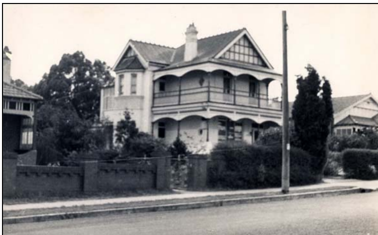
Figure 2.4 c. 1964 photograph showing that the building had been painted by this time. Part of the original two storey section of the original rear wing is also just visible.
