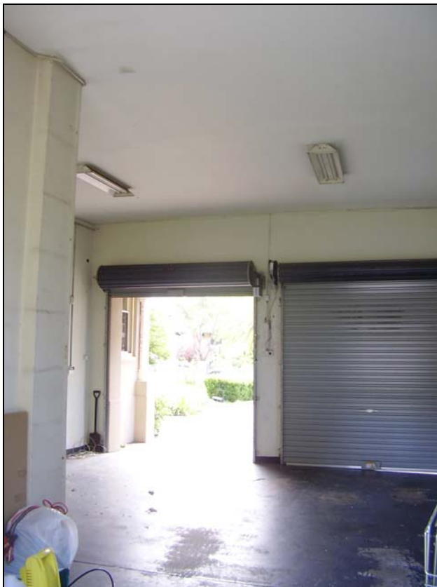
Figure 3.55 The garage on the ground floor of the rear wing is simply finished with concrete floor slab, painted masonry walls and flat ceiling with surface mounted lighting.
