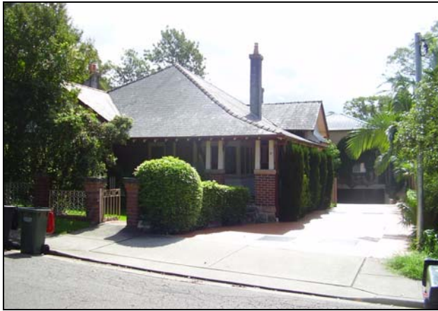
Figure 3.19 No. 27 Wyatt Avenue is a single storey Federation period house with hipped and gabled roof clad in slates and open front verandah. The building retains its street presence despite the addition of a stencilled concrete driveway and modern residential development at the rear.
