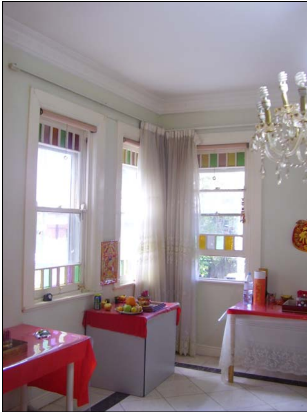
Figure 3.54 The rear wing generally incorporates modern fabric and linings, however, it would appear some original windows may have been reused on the front façade.
