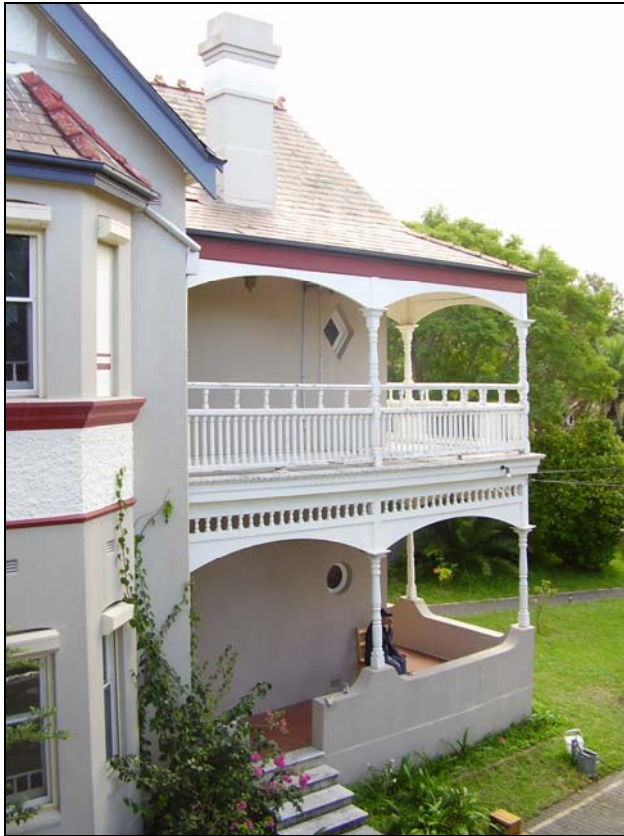
Figure 3.31 The front main wing also retains original east facing gable and faceted bay with rendered and rough cast details and hipped roof over.
