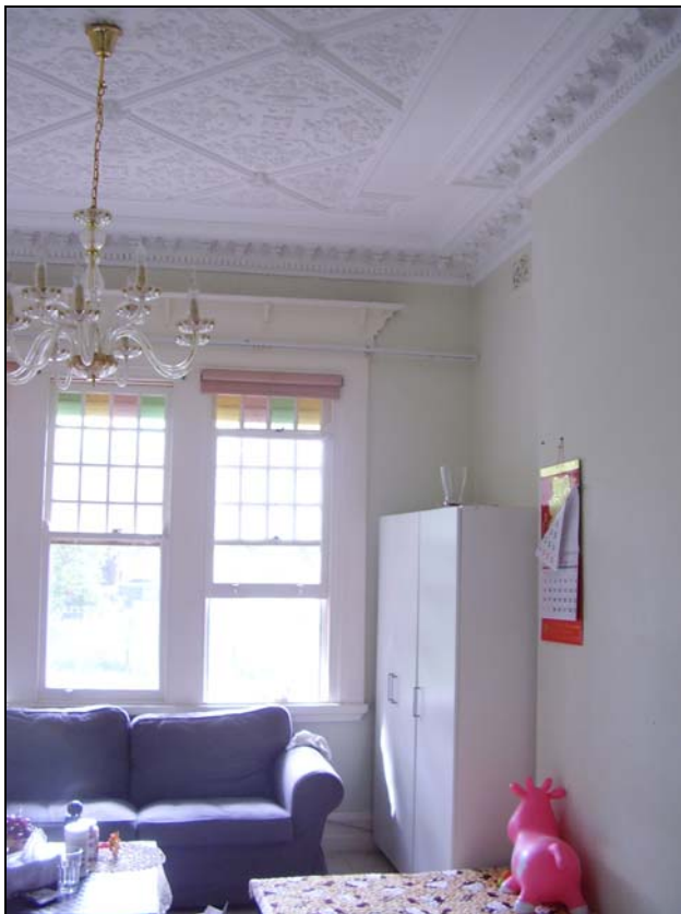
Figure 3.45 The front ground floor sitting room also retains a chimney breast, however, the fireplace has been infilled and surround previously removed.
