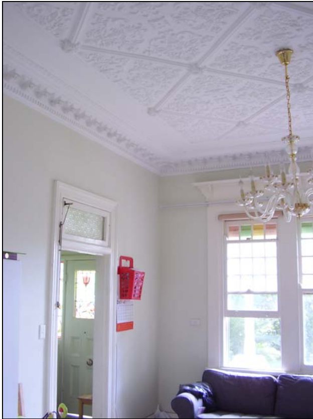
Figure 3.44 The front, ground floor room retains original richly decorated ceiling and timber joinery including timber windows and architrave on the northern wall.
