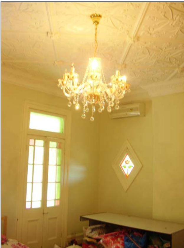
Figure 3.49 The front room on the first floor of the main, original wing also retains the original decorative plaster ceiling and coving, also wall vents, chimney breast, small feature window and French doors accessing the front balcony.
