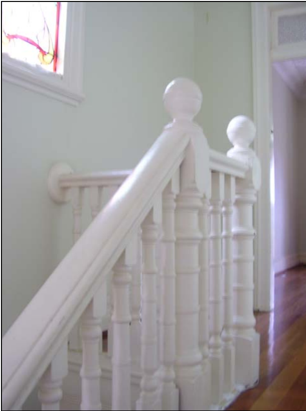
Figure 3.48 The stair balustrade and upper landing. The timber floors throughout appear to have been replaced.
