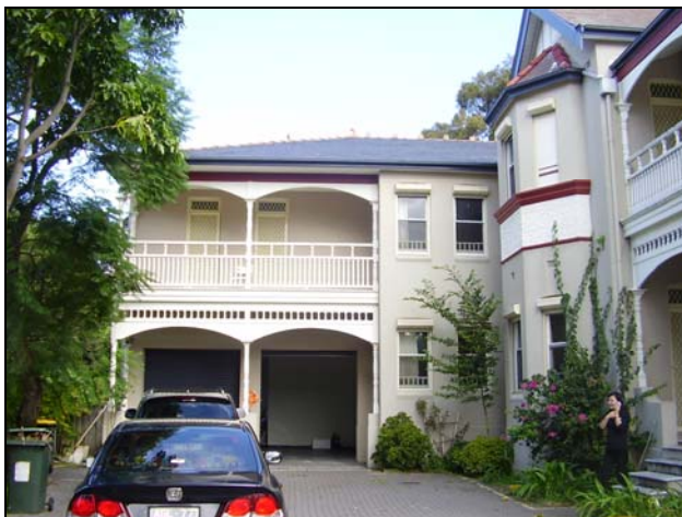
Figure 3.33 The “rear” wing constructed in the late 1980s has garage openings on the ground floor with open balcony over. The hipped roof has modern slate tiles to reflect the original with terracotta trims. The balcony and garage openings have modern timber elements that have been detailed to match the original verandah and balcony details. The windows may have been recycled from the demolished original rear wing or fabricated to match original windows.
